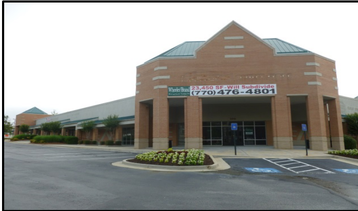
Before – blighted and obsolete
