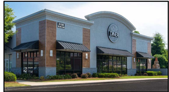
After – renovated outparcel
